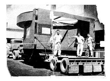
Generally, there are three basic steps in order to move a structure: first it is important to prepare the home to be independent from its foundations (see illustration 8). After the house becomes an independent object the structure is set upon temporary foundations (see illustration 9). The final step is to set the structure's loads upon the truck . (See illustration 10)
